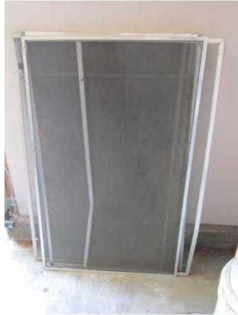
Photo 43 Two of these appear usable. Note: these types of screens can also be repaired.
