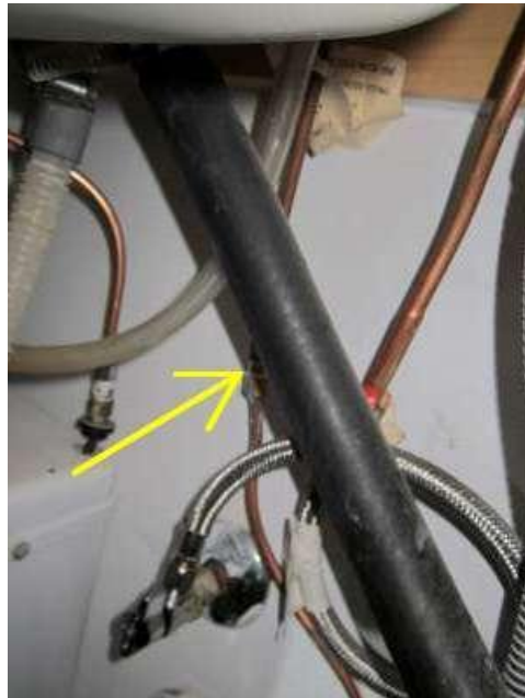
Photo 38 Leak source.
